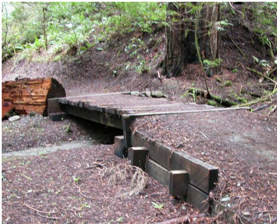
Photo 26.8 - Maintained Puncheon
