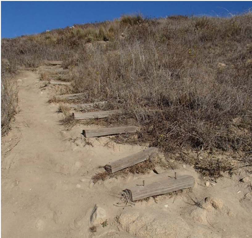
Photo 26.11 - Step Carriage in Need of Replacement
