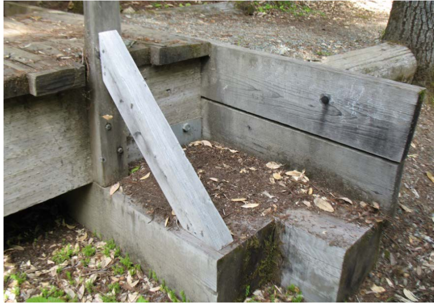
Photo 26.5 - Bridge Stringer (good air gap) and Mudsill (organic buildup)
