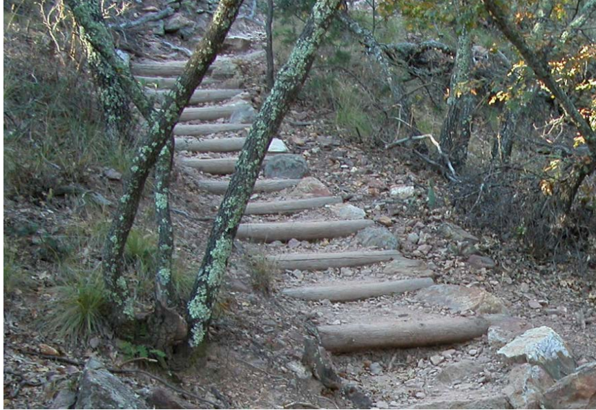
Photo 26.12 - Steps in Need of Tread Maintenance
