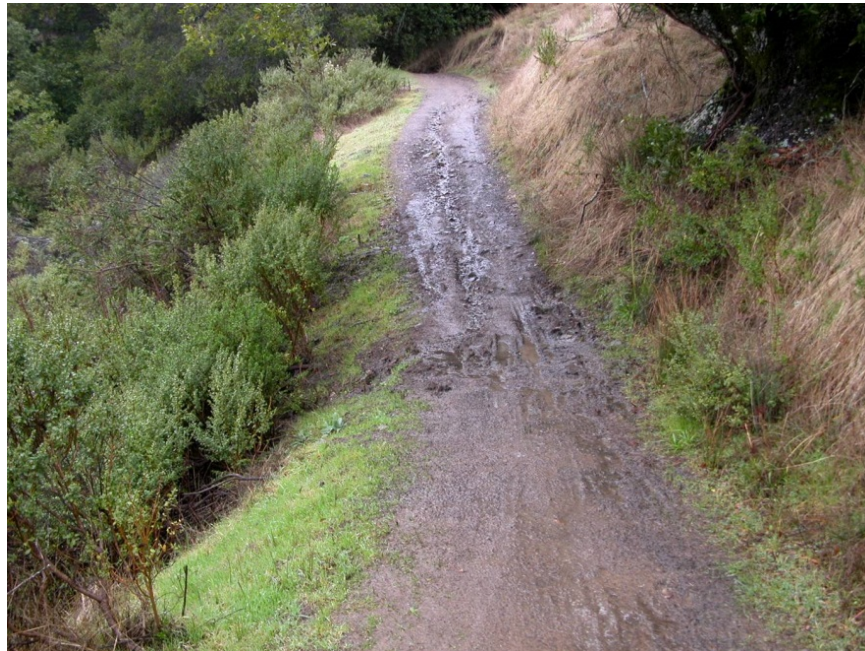
Photo 26.4 - Unmaintained Drain Dip
