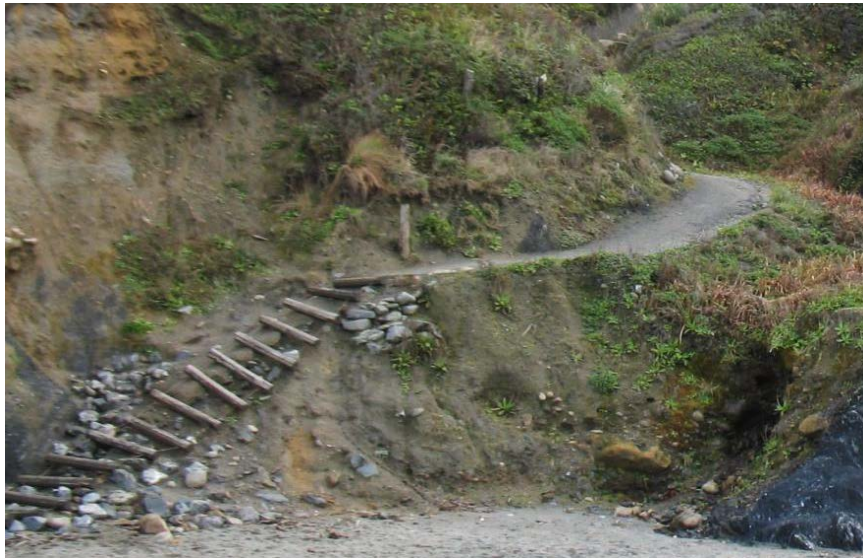
Photo 26.13 - Cable Steps in Need of Reset
